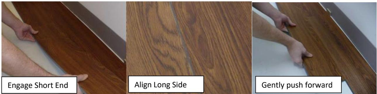
8. Continue working from left to right maintaining the random appearance. Planks may be installed row by row or by working multiple rows using the stair step method. Be sure to maintain proper spacing at walls and vertical obstructions
