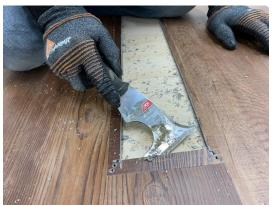
8. Prepare the replacement plank by removing the tongue and groove on each short side and by removing the groove on the long side.
