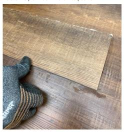
14. Roll seam edges with a hand roller to ensure proper contact with floating seam tape.
