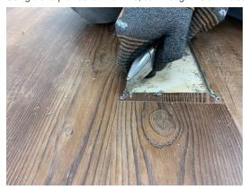
7. Carefully remove the edges of the cut plank. Do not damage adjoining planks.
