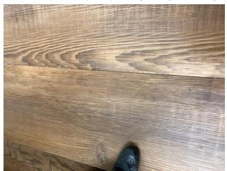
13. Rotate the plank downward into position.
