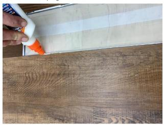
12. Position the replacement plank by inserting the tongue of the long side into the groove of the adjoining plank.
