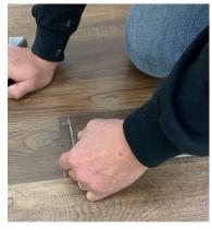
5. Using a power drill with a 1/8" bit, drill from each corner back to the inside edge. Space the holes approximately 1/16".
