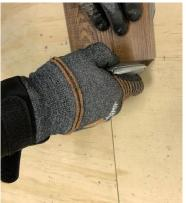
9. Using Tarkett S 875 Floating Seam Tape, place a piece so it is centered under each adjoining plank. Use a handroller to ensure proper bond.
