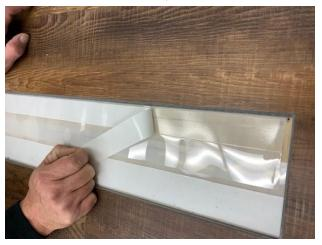
11. Place a bead of PVA adhesive (similar to Elmer's Glue All) on the top of the tongue of the adjacent plank, long and short side. Wipe off the excess with a damp rag.
