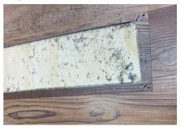
6. Using a sharp chisel or lino knife, cut through the drill holes.
